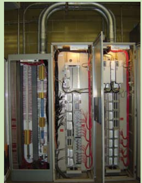
One of the numerous Interface Termination Units (ITCs) on site at Blue Plains linking processes to PCS.
